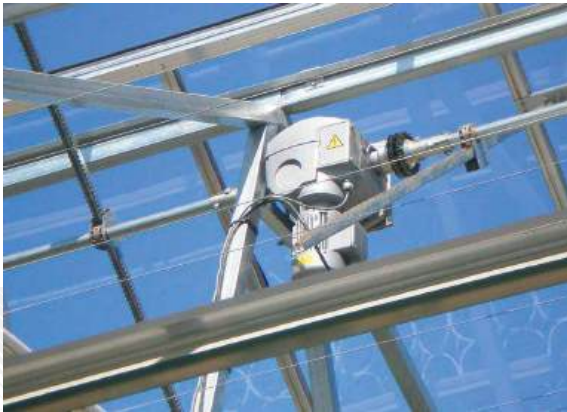
Example of Open-Roof ventilation with Type A
